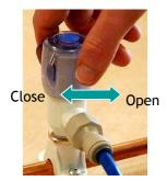
1. Locate the shut-off valve and turn off the mains water supply to the filter housing.
