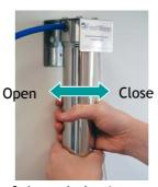
3. Leave the housing assembly on the bracket. Firmly grip the sump with both hands and turn to the left to release the seal. The sump of the filter will be full of water so position the bowl carefully to catch the residual water.
